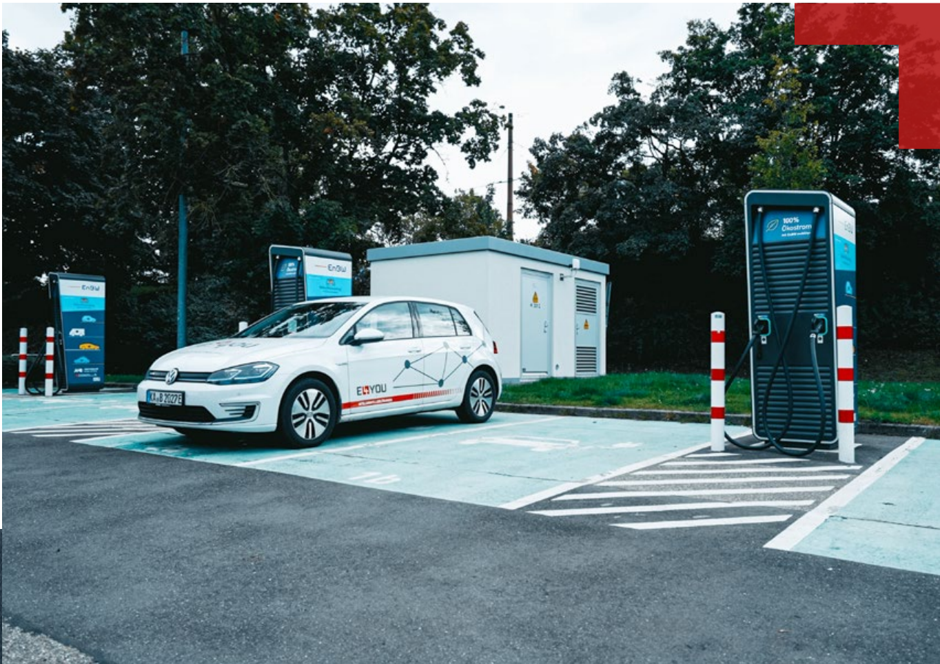
Compact Substation in public area for supplying electricity to a charging point
